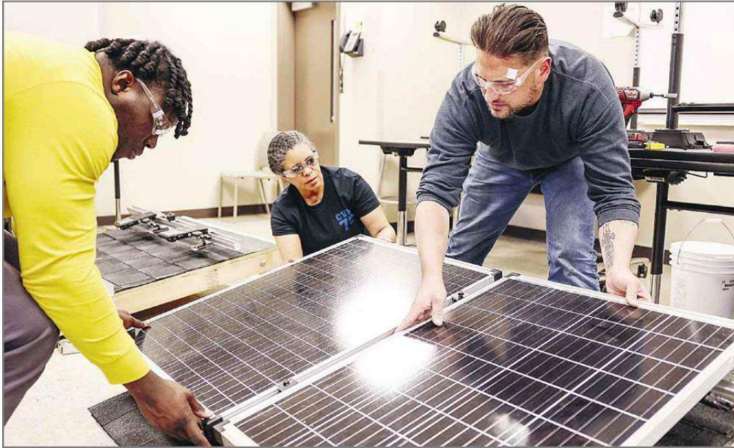
Students learn to attach solar panels to roofs in the SCCC solar technology program in Brentwood.
